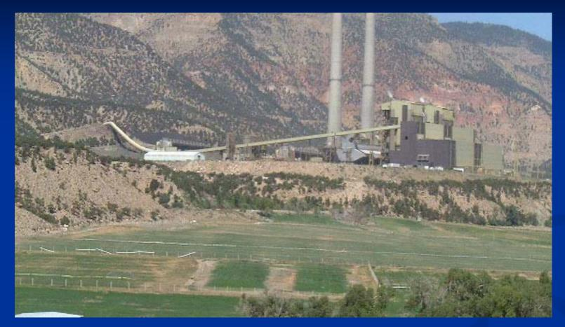
Power plant has zero discharge permit for spent cooling water.
